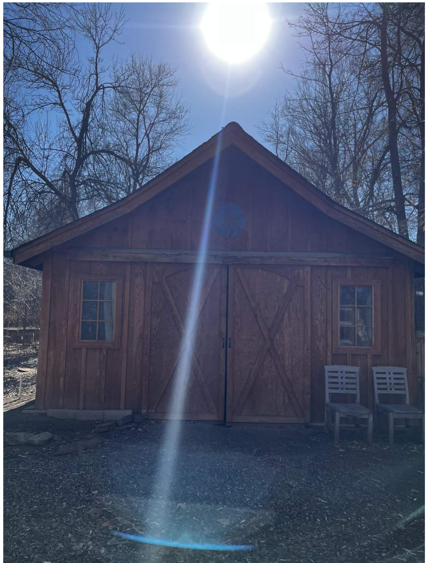
EXISTING STRUCTURE: SHED Photos: February 2025
