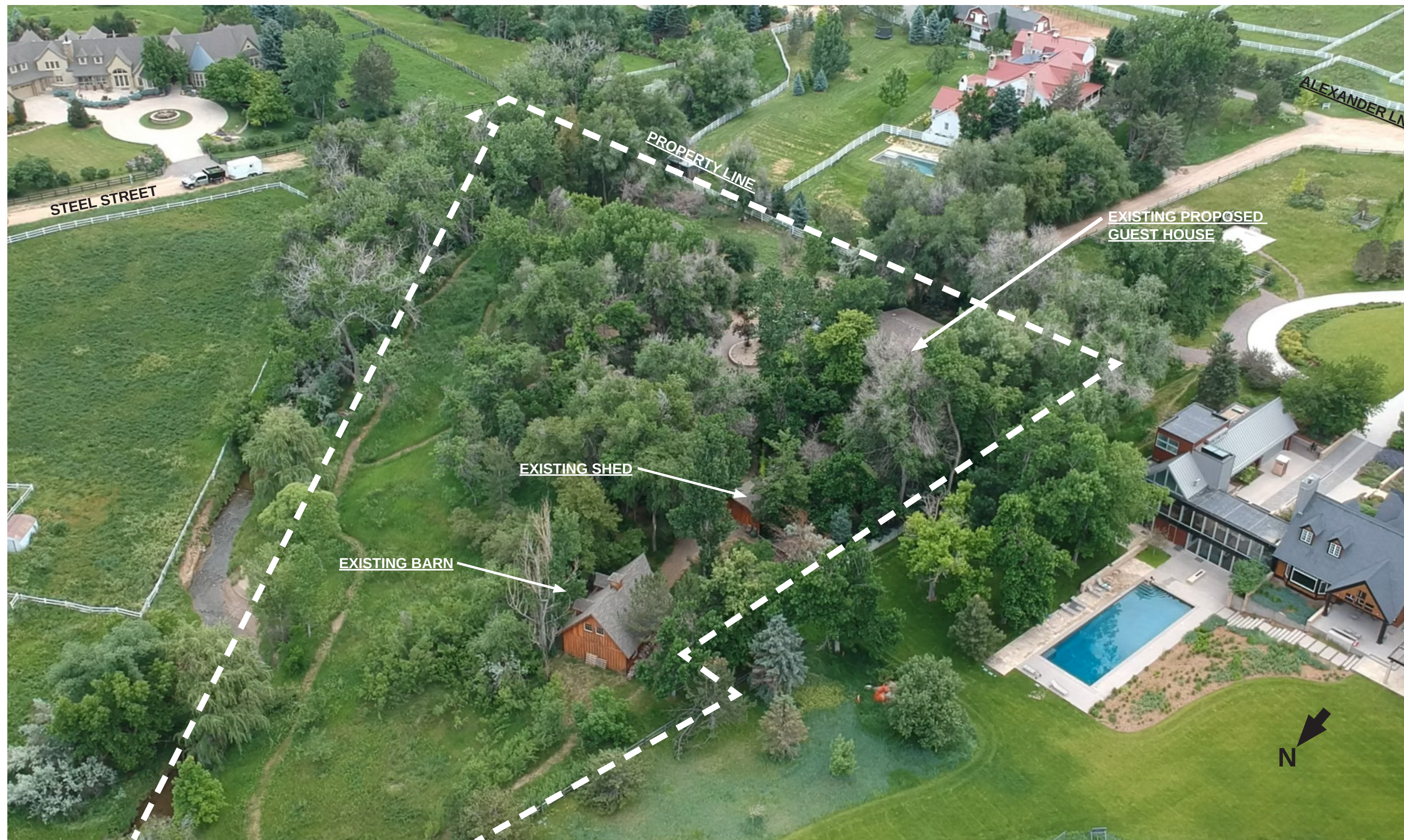
SITE AERIAL FROM NORTH WEST
